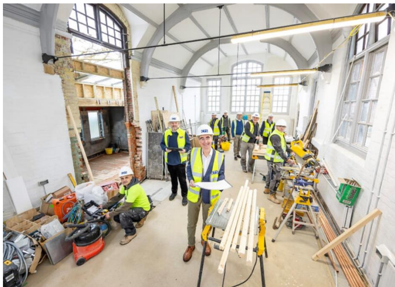
Figure 25: Final construction stage Twyford Library
