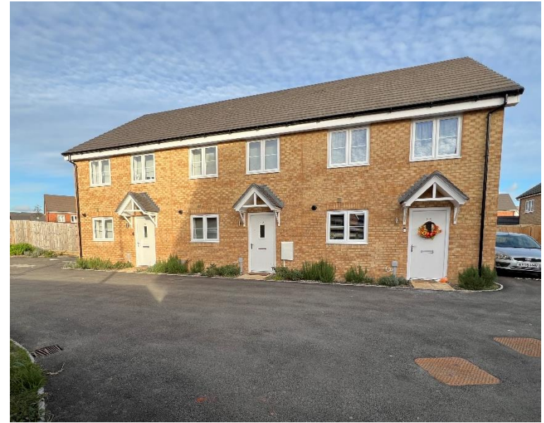
Figure 44: Shinfield West Terraces. Delivered by Bovis.
