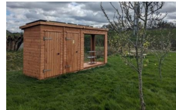
Figure 31: Solar Panels at Winnersh Allotments
