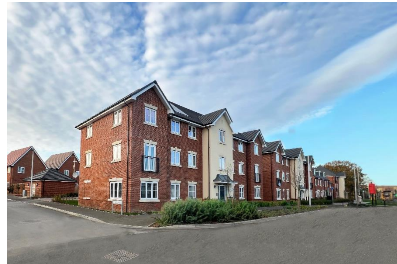
Figure 41: Finchwood Park. Delivered by Legal and General.
