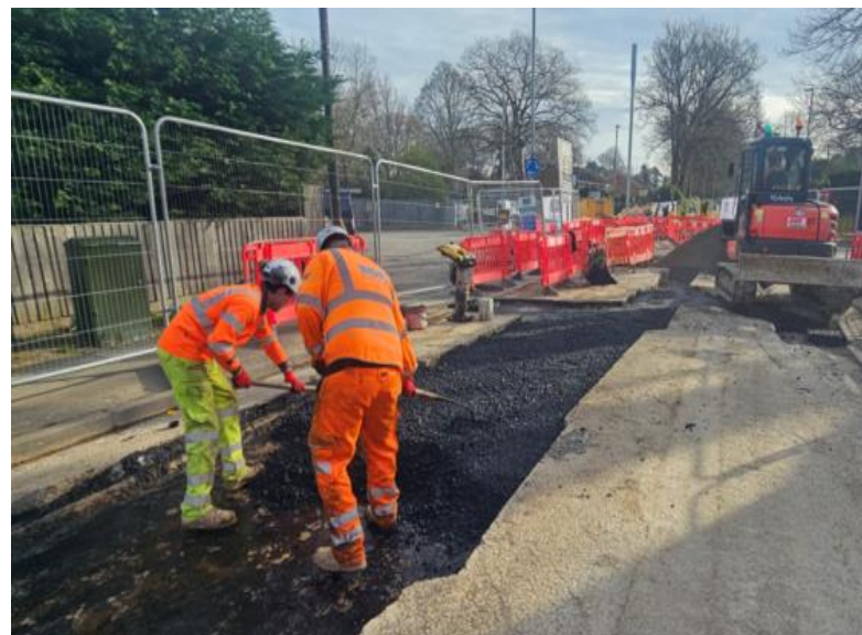
Figure 19: California Crossing Improvement works
