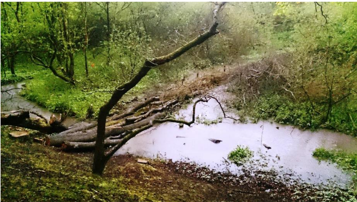
Figure 11.5 Example of a leaky dam
